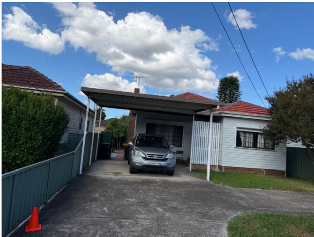
Figure 1 – 215 The River Road, Revesby – 1 storey Dwelling – Existing Vinyl Cladding Residence with tiled roof
