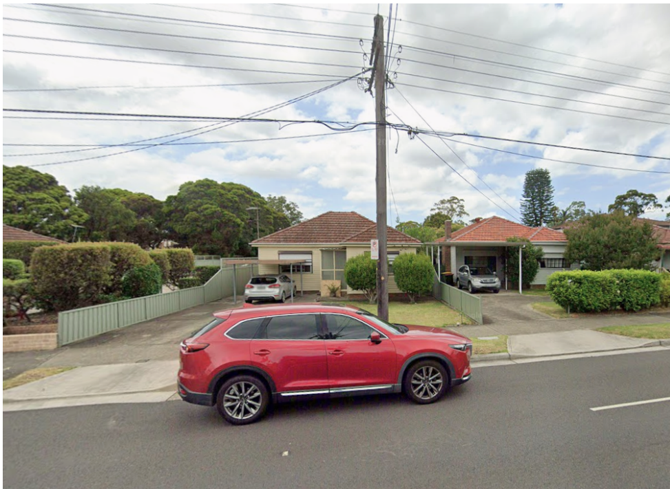
Figure 3 – 213 The River Road, Revesby– 1 storey Dwelling – Existing Cladding Residence with tiled roof
