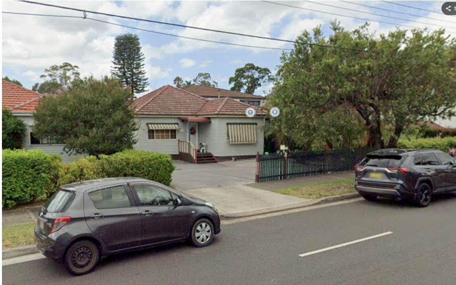
Figure 2 – 217 The River Road, Revesby – 1 storey Dwelling – Existing Cladding Residence with tiled roof
